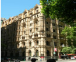
FORMER NATIONAL MUTUAL LIFE ASSOCIATION BUILDING SOHE 2008
