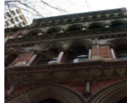
south australian insurance building collins street melbourne front elevation sep1999
