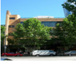
FORMER MCPHERSONS BUILDING SOHE 2008
