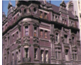
melbourne city building elizabeth street melbourne front detail feb1978
