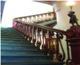
Art Gallery post restoration 2010
