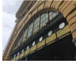
FLINDERS STREET RAILWAY STATION COMPLEX October 2016
