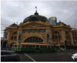
FLINDERS STREET RAILWAY STATION COMPLEX October 2016
