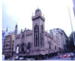
h00438 1 forum theatre flinders street melbourne external view she project 2003
