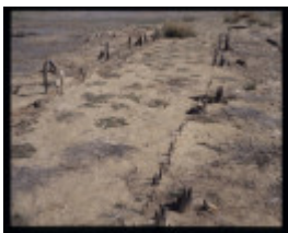
LAKE BOORT DAM
