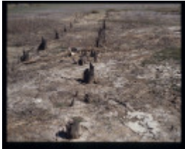
LAKE BOORT DAM
