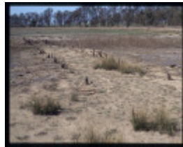
LAKE BOORT DAM
