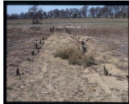
LAKE BOORT DAM
