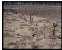
LAKE BOORT DAM
