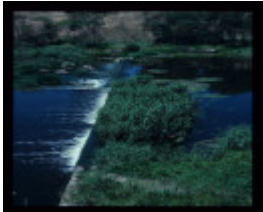
BUCKLEYS FALLS PUMPING STATION
