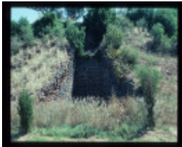
OLD STEIGLITZ ROAD BRIDGE
