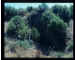
OLD STEIGLITZ ROAD BRIDGE
