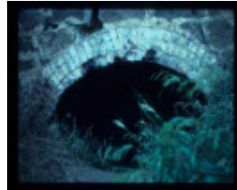
OLD STEIGLITZ ROAD BRIDGE FEATURE
