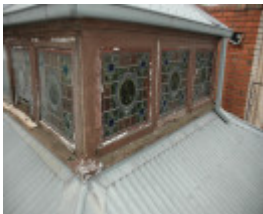
Before Photograph - Reference F3907 2014
