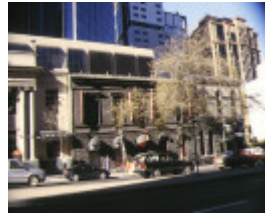
1 former levicks & piper wholesale ironmonger's warehouse king street melb front view
