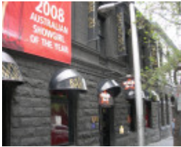
FORMER LEVICKS AND PIPER WHOLESALE IRONMONGERS WAREHOUSE SOHE 2008
