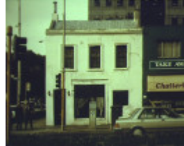
1 building 330 king street front view
