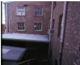
former phoenix clothing company king street melbourne side view rear windows
