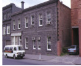
1 langdon building king street melbourne front view
