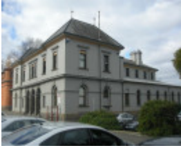
Building F, Former Supreme Court.jpg
