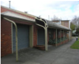
Building H and I, Corbould Building, Automotive Skills Centre.jpg
