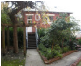
Building O, Old Plumbing Building.jpg
