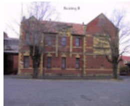
h01463 school of mines lydiard street south ballarat arts bldg b
