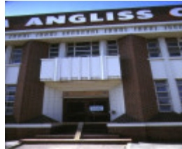
william angliss college la trobe street melbourne front entrance feb1985
