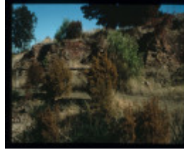
CALEDONIAN CRUSHING MILL
