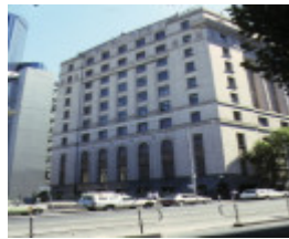
former port of melbourne authority building market street melbourne side view mar1980
