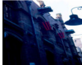
h00473 warehouse niagara lane
