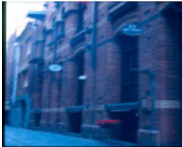
h00473 warehouses niagara lane3
