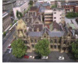
1 magistrates court russell street melbourne aerial view
