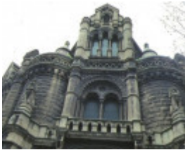
magistrates court russell street melbourne entrance elevation
