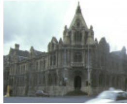
magistrates court russell street melbourne front view
