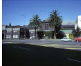
1 old melbourne gaol russell street melbourne front view jan1979
