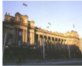
1 parliament house grounds works & fences spring street melbourne front view
