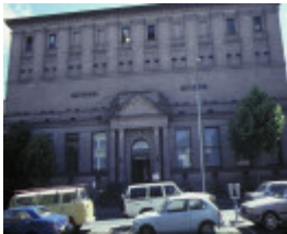
state library of victoria & national museum complex museum entrance russell street jan1985
