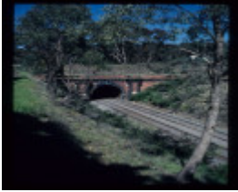
ELPHINSTONE RAILWAY TUNNEL
