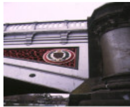
princes bridge over yarra river melbourne side detail
