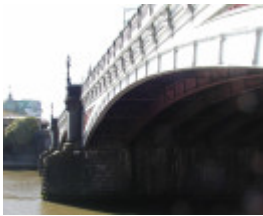
h01447 princes bridge st kilda road over yarra river melbourne below she project 2004
