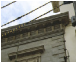
anz bank ballarat roof detail
