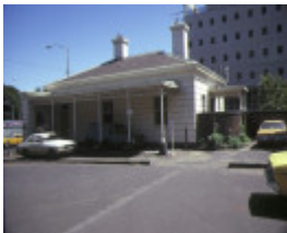
former royal mint williams street melbourne caretaker's cottage feb1985
