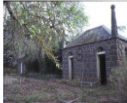
exford homestead exford street melton south bluestone outbuilding apr1980
