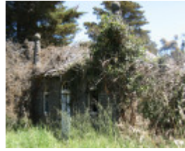
Exford west pavilion
