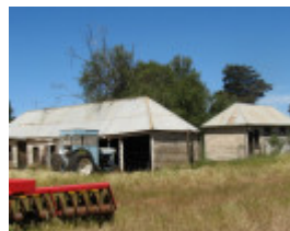
Exford stable buildings
