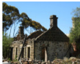
Exford blacksmith forge & residence
