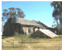
Exford barn & underground tank
