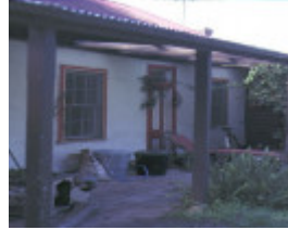
koonoona merricks road merricks north detail of front verandah aug1982
