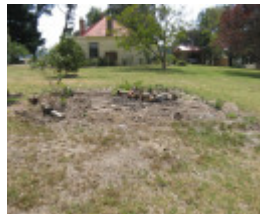
Koonoona Merricks Road Merricks north Unauthorised demolition of wood shed
