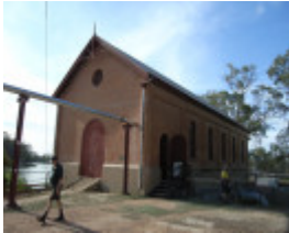
PSYCHE BEND PUMPING STATION SOHE 2008
