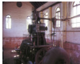
psyche bend pumping station psyche bend mildura interior with machinery
