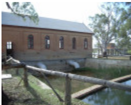
PSYCHE BEND PUMPING STATION SOHE 2008
