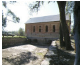
1 psyche bend pumping station psyche bend mildura rear view
