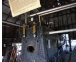
PSYCHE BEND PUMPING STATION SOHE 2008
