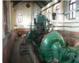
PSYCHE BEND PUMPING STATION SOHE 2008
