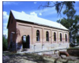
psyche bend pumping station psyche bend mildura front view dec1990
