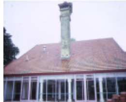
walter burley griffin incinerator holmes rd moonee ponds side view sep1985
