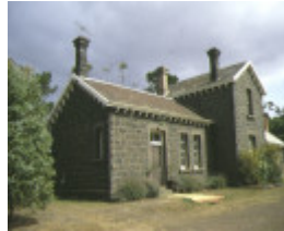
former moorabool railway station front view dec1998
