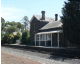
FORMER MOORABOOL RAILWAY STATION SOHE 2008
