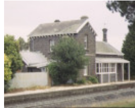
1 former moorabool railway station platform view dec1998
