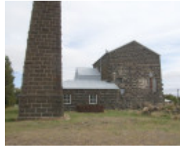
CHIMNEY & BLUESTONE MILL SOHE 2008
