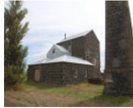
CHIMNEY & BLUESTONE MILL SOHE 2008
