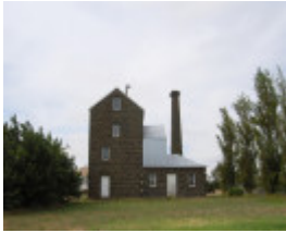
CHIMNEY & BLUESTONE MILL SOHE 2008
