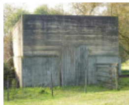
Concrete silage store from west 2017.jpg
