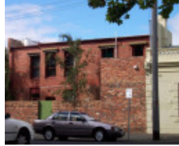
Rear of 366 Rathdowne Street.JPG
