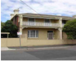
richmond waltham street richmond waltham street 39
