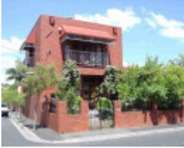
richmond wangaratta street richmond wangaratta street 1
