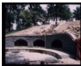
FORMER GOVERNMENT CAMP PRECINCT (ROSALIND PARK) EXCAVATION
