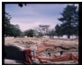
FORMER GOVERNMENT CAMP PRECINCT (ROSALIND PARK) EXCAVATION
