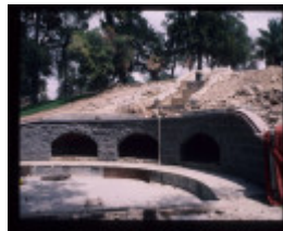
FORMER GOVERNMENT CAMP PRECINCT (ROSALIND PARK) EXCAVATION
