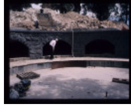
FORMER GOVERNMENT CAMP PRECINCT (ROSALIND PARK) EXCAVATION
