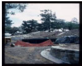
FORMER GOVERNMENT CAMP PRECINCT (ROSALIND PARK) EXCAVATION
