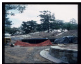
FORMER GOVERNMENT CAMP PRECINCT (ROSALIND PARK) EXCAVATION
