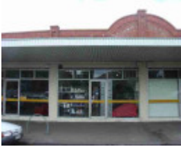
carlton north park street carlton north park street 324
