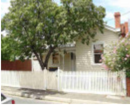
richmond tyson street richmond tyson street 13
