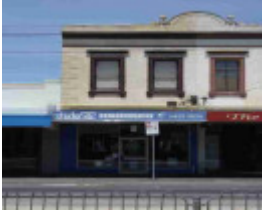
burnley bridge road burnley bridge road 502
