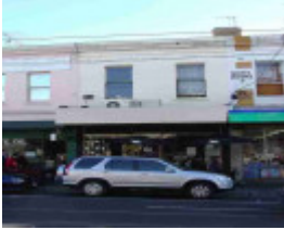
cremorne church street cremorne church street 460
