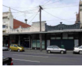
Collingwood Johnston Street 105-113.JPG
