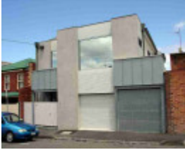
richmond dando street richmond dando street 4
