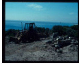
FORT NEPEAN GUN EMPLACEMENT EXCAVATION
