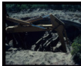
FORT NEPEAN GUN EMPLACEMENT EXCAVATION
