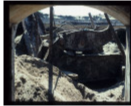
FORT NEPEAN GUN EMPLACEMENT EXCAVATION
