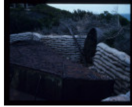
FORT NEPEAN GUN EMPLACEMENT EXCAVATION
