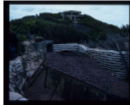
FORT NEPEAN GUN EMPLACEMENT EXCAVATION
