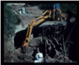
FORT NEPEAN GUN EMPLACEMENT EXCAVATION
