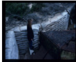
FORT NEPEAN GUN EMPLACEMENT EXCAVATION
