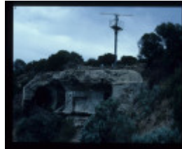
FORT NEPEAN GUN EMPLACEMENT EXCAVATION
