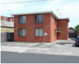
collingwood bendigo street collingwood bendigo street 17-15 unit 1
