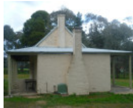
Before Photograph - Reference F3875 2014
