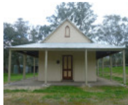
Before Photograph - Reference F3875 2014
