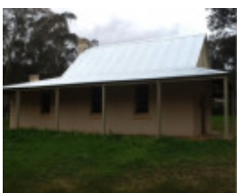
After Photograph - Reference F3875 2016
