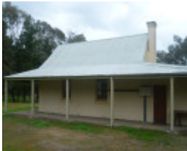
Before Photograph - Reference F3875 2014
