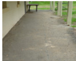
Before Photograph - Reference F3875 2014
