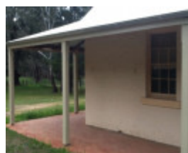
After Photograph - Reference F3875 2016
