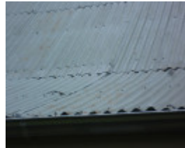
Before Photograph - Reference F3875 2014
