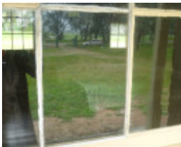
Before Photograph - Reference F3875 2014
