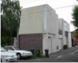
richmond brighton street richmond brighton street 146
