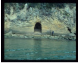
QUARANTINE STATION LIME KILN 1
